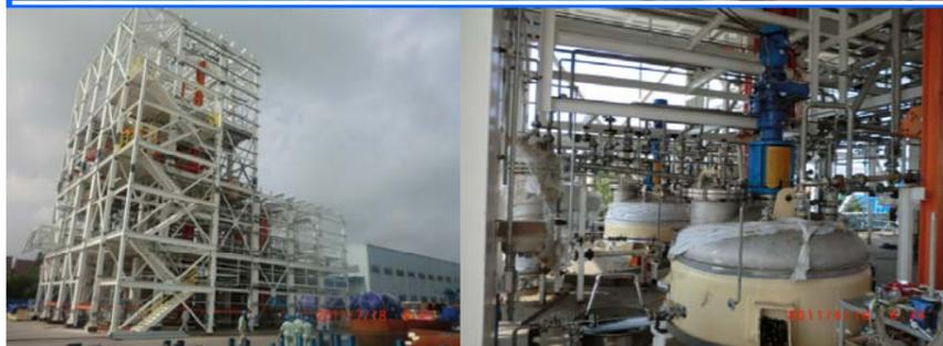
This is a chemical plant modular project in Saudi Arabia. MHI's work scope covers fabrication, coating, packing, full trial assembly in Changshu, China and delivery. MHI finished the full assembly for 36 large modules in total with it's rich experience in handling and lifting. The largest modular is 10 tons with a height of 12m. MHI has presented a tread to focus on large modular project recently while it's ability to handle modular project has become mature.
